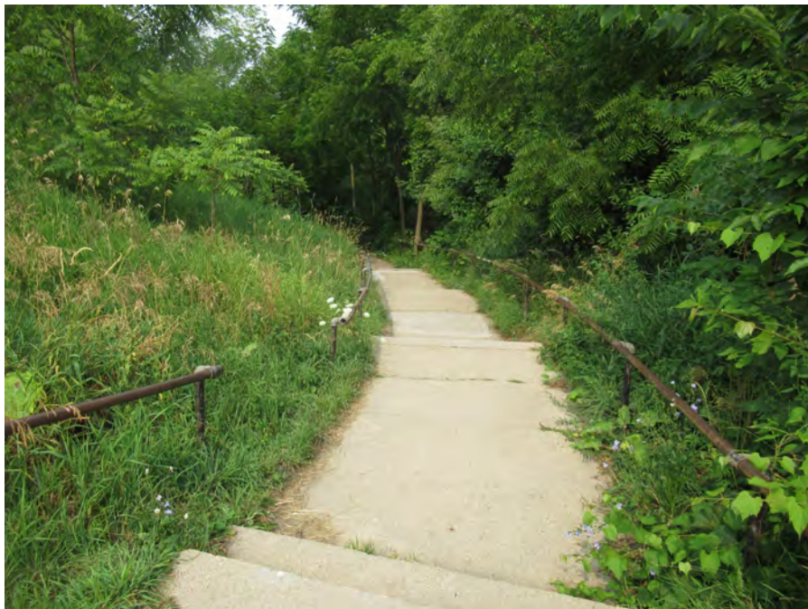
The switchback staircase (photo by Dan Collins)
